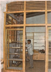
Workers at the hotel building in the City of Palaces
